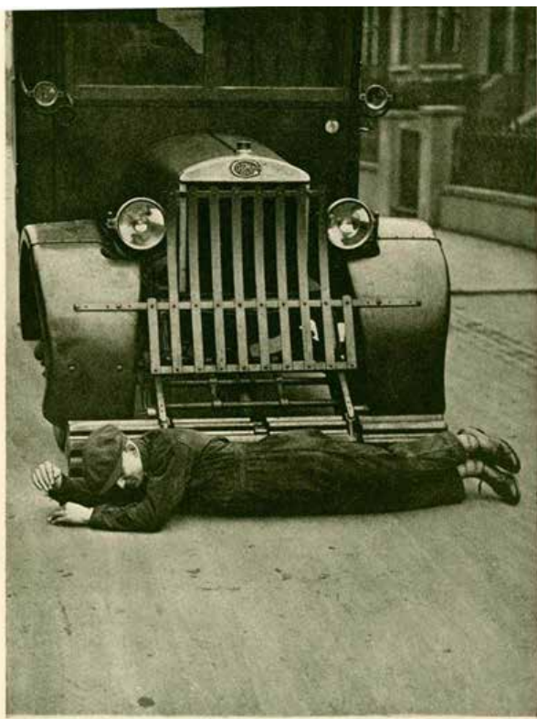
A "MAN-CATCHER." This safety device consists of three rollers attached to the radiator of the vehicle. Directly the rollers touch an obstacle, they automatically drop to the ground and push it away.
